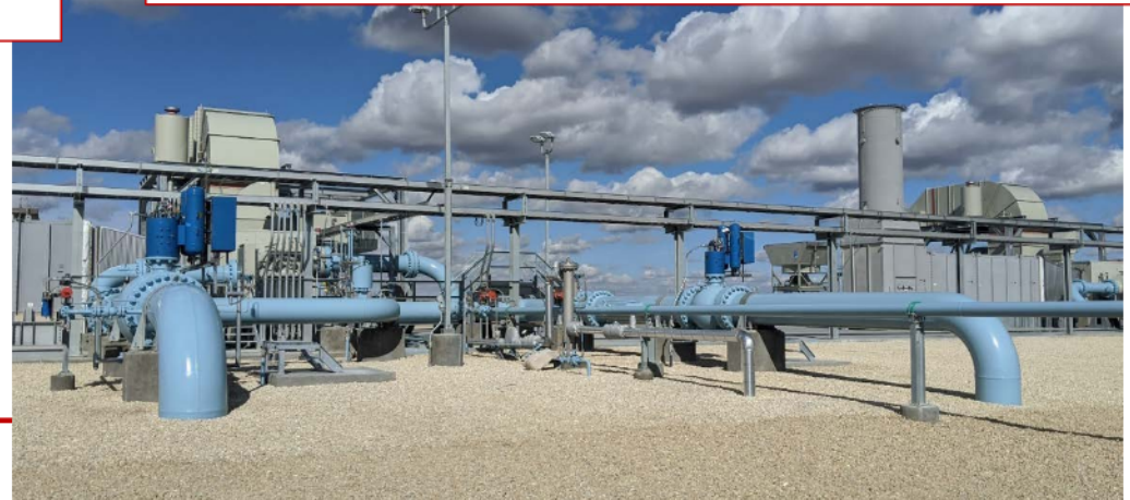
KM Midstream Examples: GCX Solar Turbines T-130 / T-250 with Enclosures / Pipeline compressors
