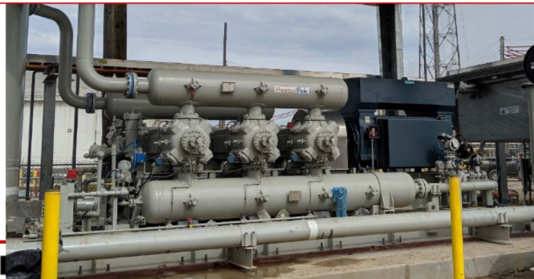
KM Midstream Examples: Ariel KBK-6 single stage unit with 4000 hp Siemens EMD packaged reliably and on time by Reagan Power
