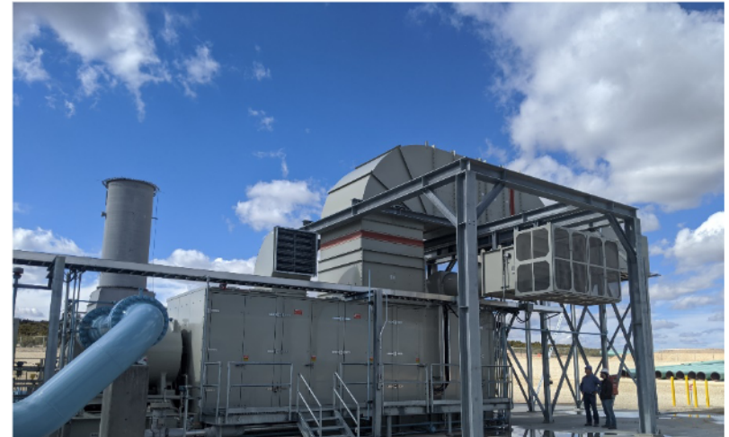
KM Midstream Examples: GCX Solar Turbines T-130 / T-250 with Enclosures / Pipeline compressors
